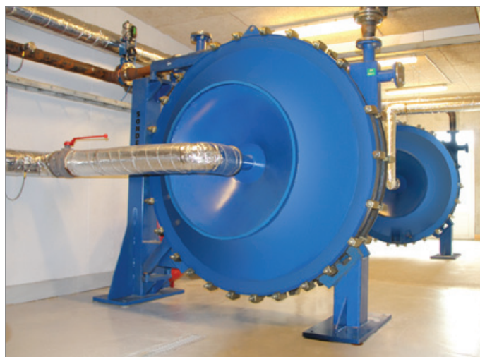
Sondex spiral heat exchanger at Linko Gas in Denmark
