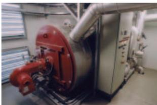
Horizontally installed heater for the food industry pre-mounted and wired as compact unit
